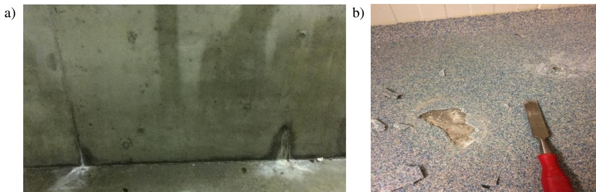
**Fig. 1. Examples of issues caused by leaking groundwater through concrete floors in underground structures including:** a – unsightly leaks, collection of water and long-term durability concerns; b – poor performance of floor coatings or covering
